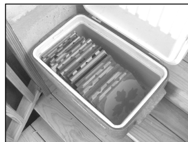
Tiles soaking in water prior to setting.
