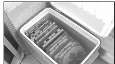
Pre-wet tiles by dipping them for 3 to 5 seconds in water prior to setting.
