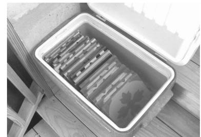
Pre-wet tiles by dipping them for 3 to 5 seconds in water prior to setting. Then letting them drip off excess in a beer cooler
